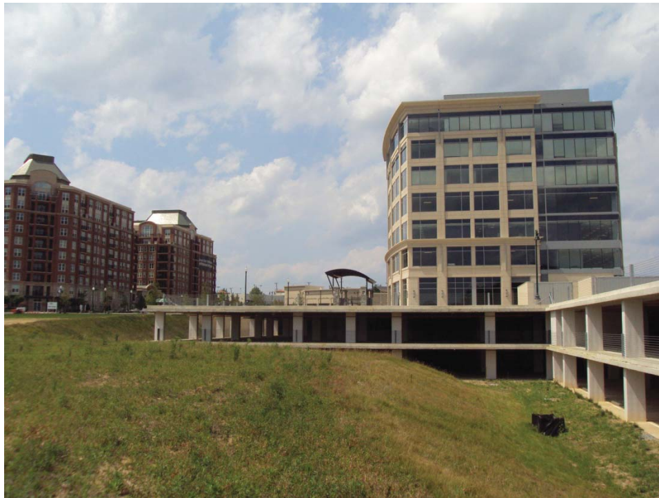
Figure 11: View from North
