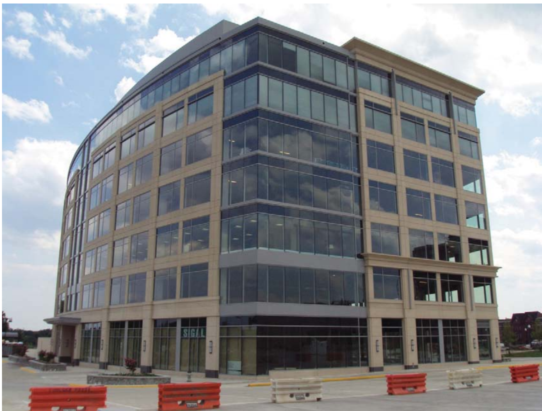
Figure 6: View of South-West Corner
